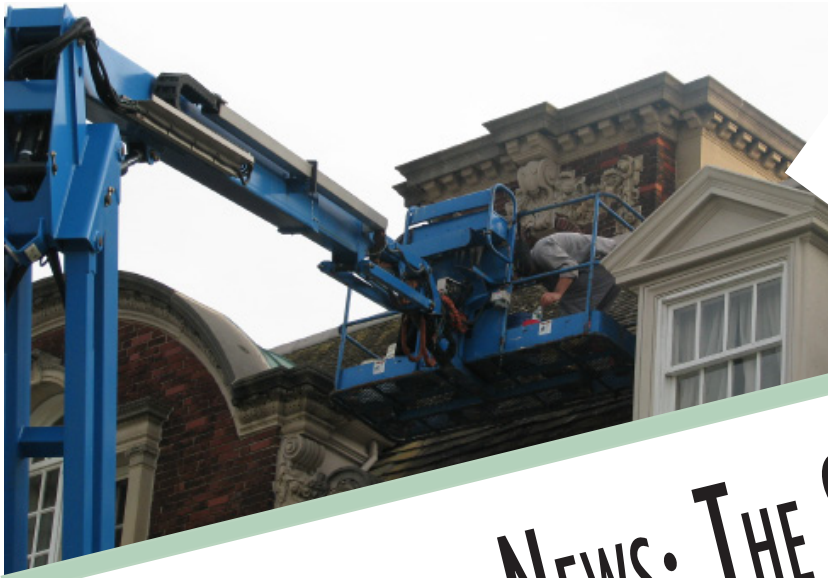
Maintenance Director, Pete DeBlasi working on the roof.
