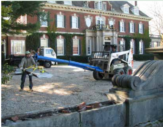
Masons rebuild the northeast section of the Westbury House courtyard wall
