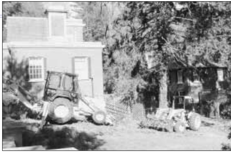
Renovating the lawn behind the servants' area of Westbury House
