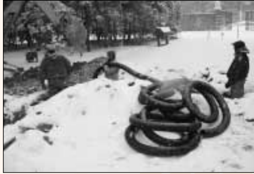
Our crew installing drainage pipe in the Garden of Appreciation
