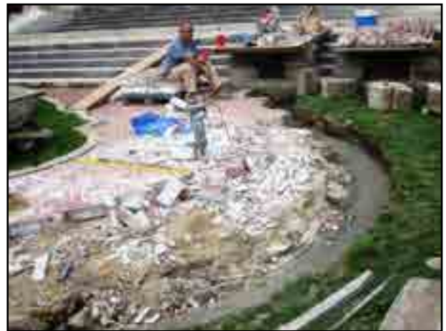
Masonry work on the South Terrace
